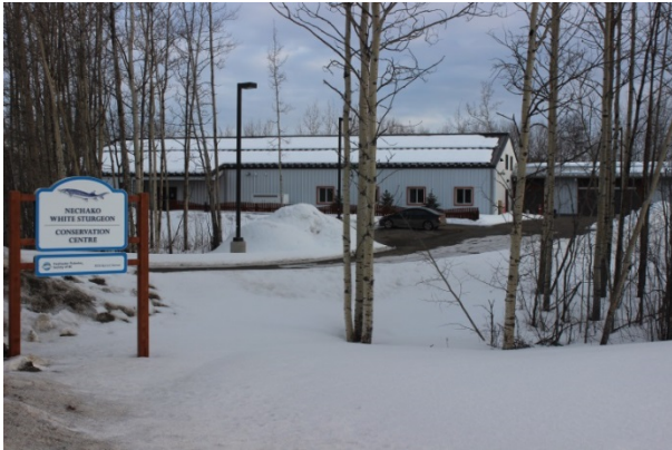
Figure 1. Completed Facility, Winter 2014
