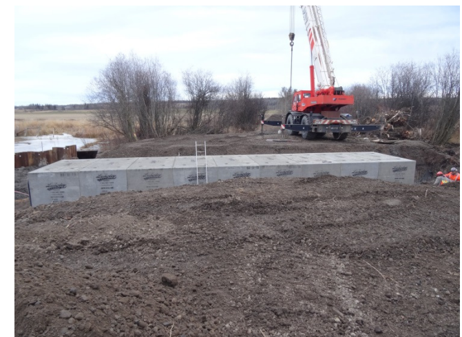
Nearing completion of new culvert placement.
