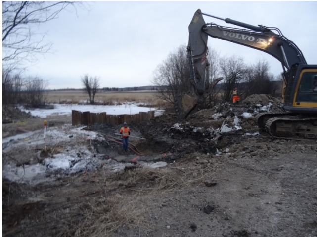
Placement of new culvert.
