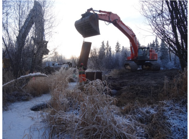
Placement of sheet piling for site isolation.
