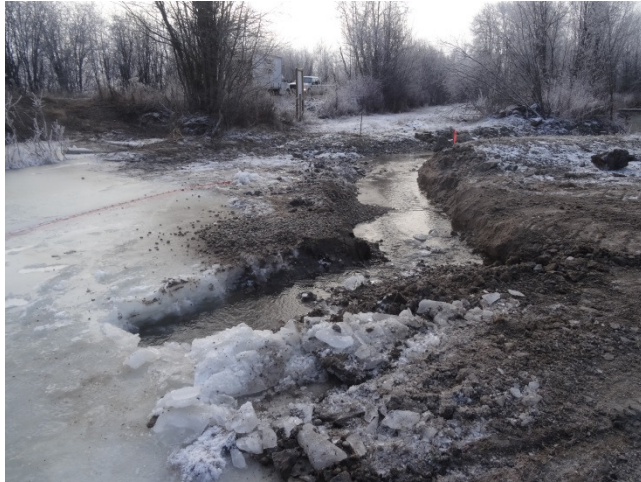
Partial diversion of existing stream into new channel.
