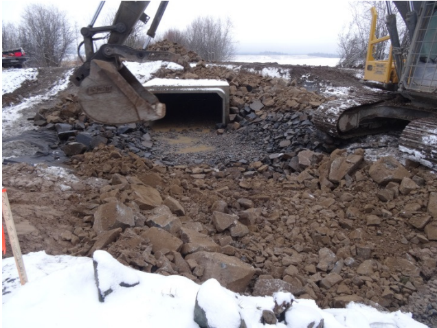
Release of water through the culvert when clean.
