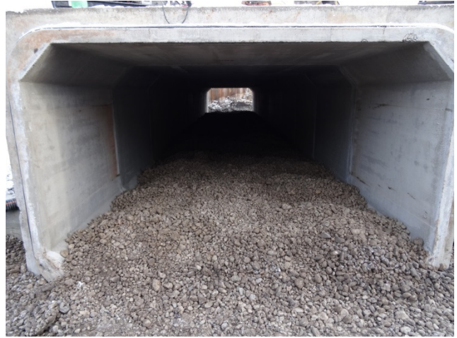
Final placement of riprap at inlet.
