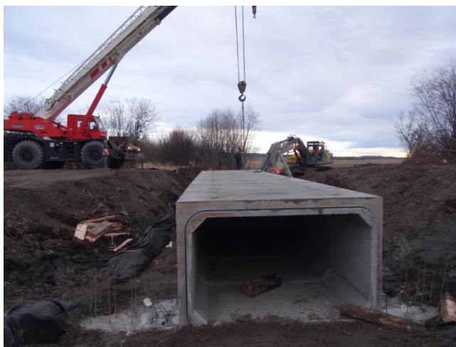
Placement of new culvert.
