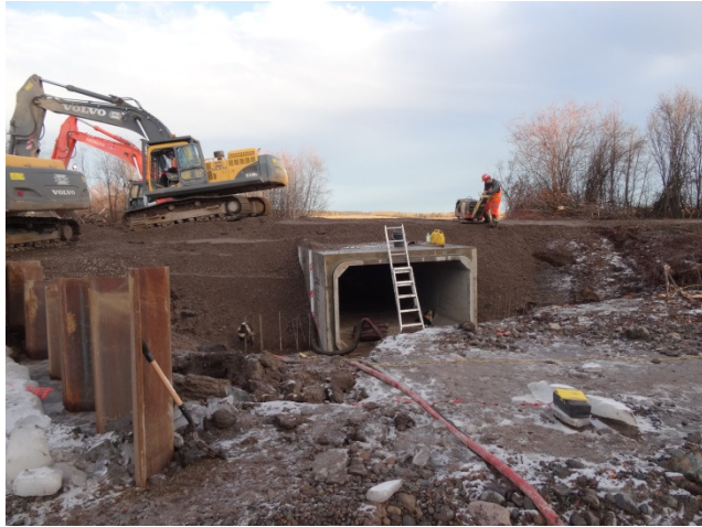
Placing and washing of riprap (outlet).
