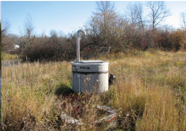
Figure 2. Pump chamber extension after completion.
