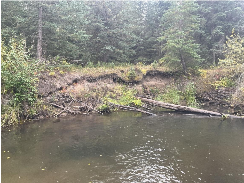
Appendix Photo D-13. Section of bank erosion observed at GR2. September 23, 2025.
