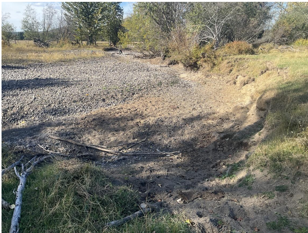
Appendix Photo D-26. Eroded banks with signs of cattle activity and vegetation clearing observed at SW1. September 24, 2025.
