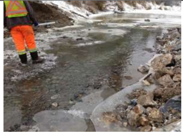
Photo 8. Stoney Creek discharge following culvert removal.
