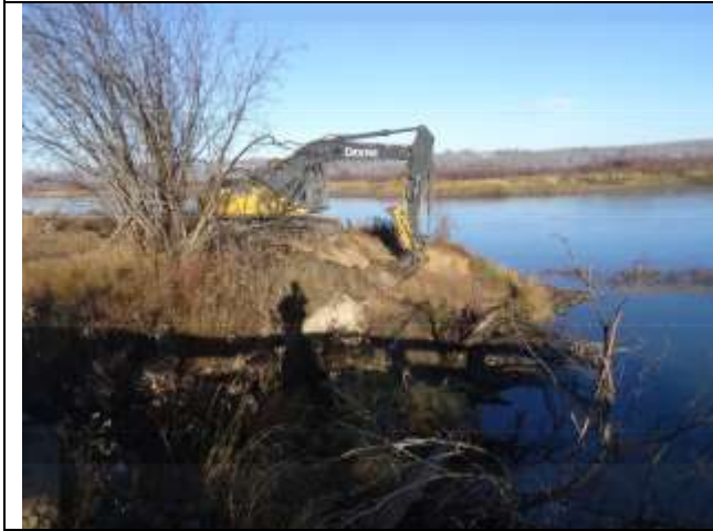
Photo 31. Re-sloping of the West bank of the mouth of Stoney Creek.
