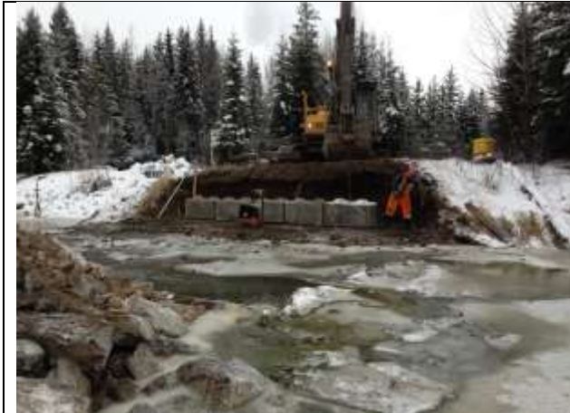
Photo 7. Post culvert removal and early stage of beam bridge installation.
