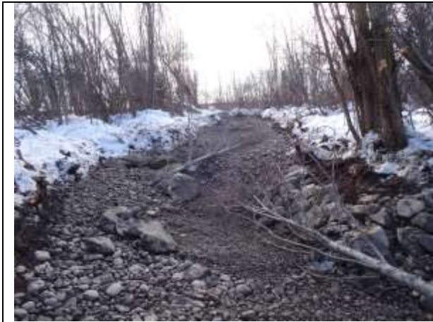
Photo 13. Felled alder trees anchored into stream channel to provide coarse woody debris habitat.
