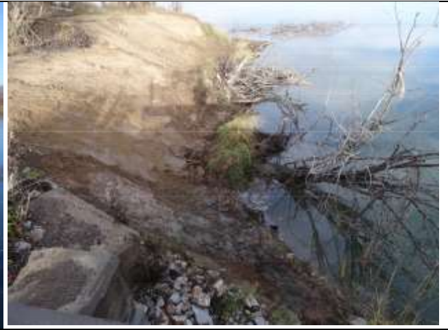
Photo 32. Re-sloped west bank of Stoney Creek prior to bank armouring and root wad placement.
