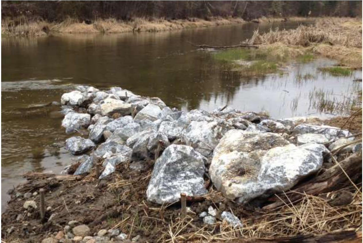
Photo 28. Willow cuttings planted within and adjacent to the V-weir upstream of the L&M Bridge, March 30, 2015. Note the extensive reed canarygrass and cattails ( Typha spp.) growing along the flood-prone channel banks - a condition characteristic of the riparian vegetation throughout lower Stoney Creek.
