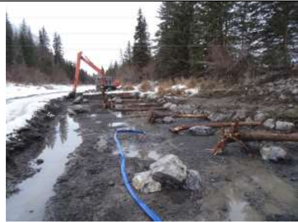
Photo 49. Root wad (LWD) and boulder clusters being added to provide fish habitat.
