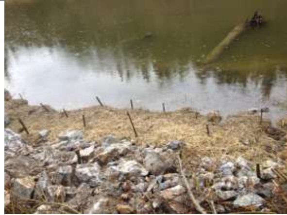
Photo 52. Willow cuttings planted below and between boulders within soft sediment at KP2+450.
