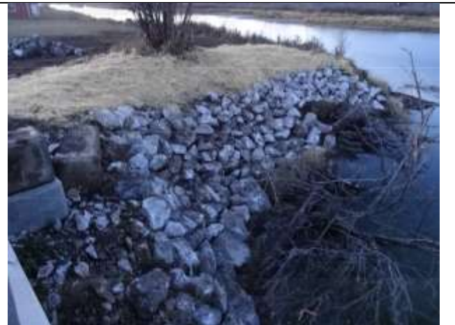
Photo 32. Re-sloped west bank of Stoney Creek prior to bank armouring and root wad placement.
