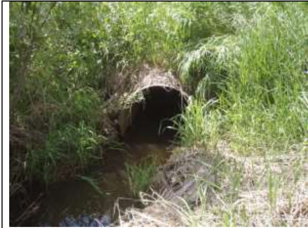
Photo 7. Inlet of main culvert at the Larson Rd crossing, June 07, 2011
