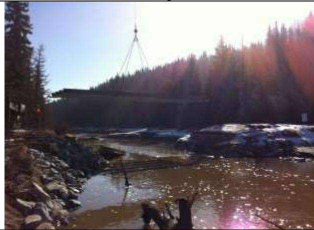
Photo 11. Beam bridge being installed on March 24, 2015 looking downstream.
