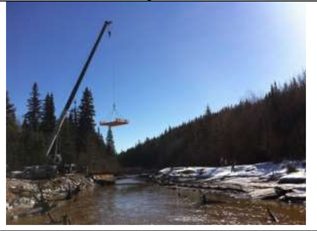
Photo 12. Latter stage of the beam bridge installation process, March 24, 2015, looking downstream.
