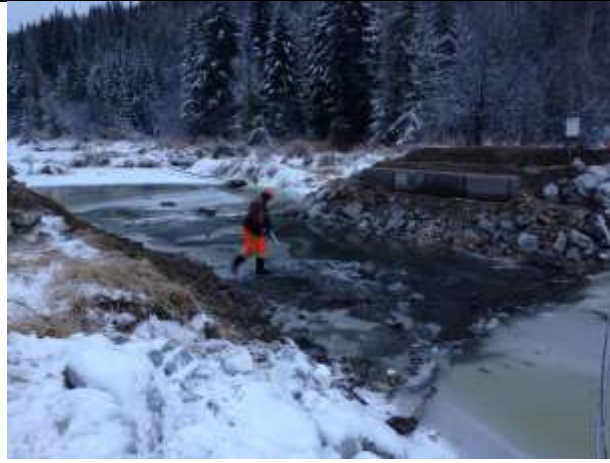
Photo 9. West beam bridge abutment.
