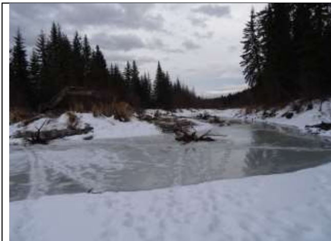
Photo 43. Boulder clusters and root wads installed on the North bank looking downstream
