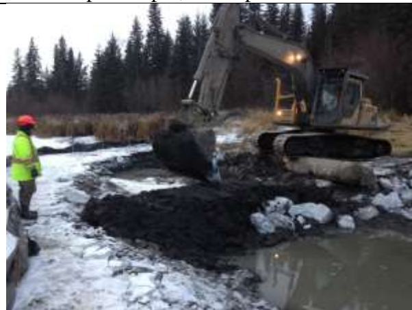
Photo 18. Installation of the V weir and channel armouring.
