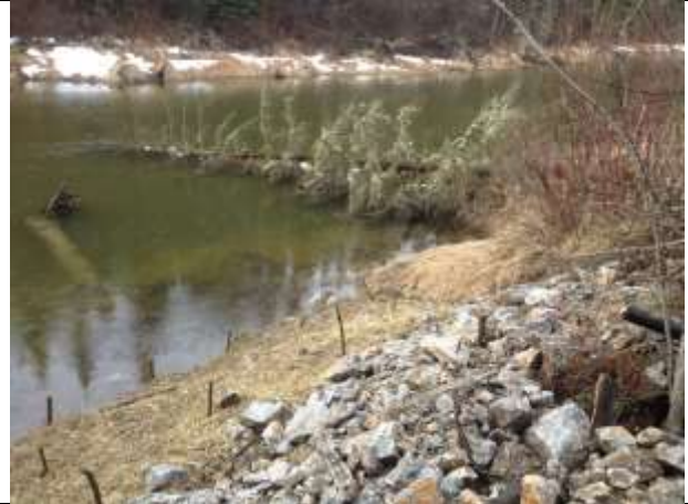
Photo 53. Willow cuttings planted at KP2+450. Note the recently fallen conifer tree.
