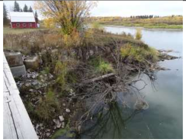
Photo 30. Stoney Creek at the Douglas Street bridge/Nechako River confluence illustrating the bank erosion occurring downstream of the bridge.
