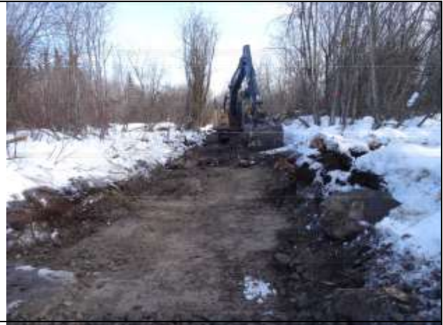
Photo 10. Reconstructing the historic channel within the alder grove.
