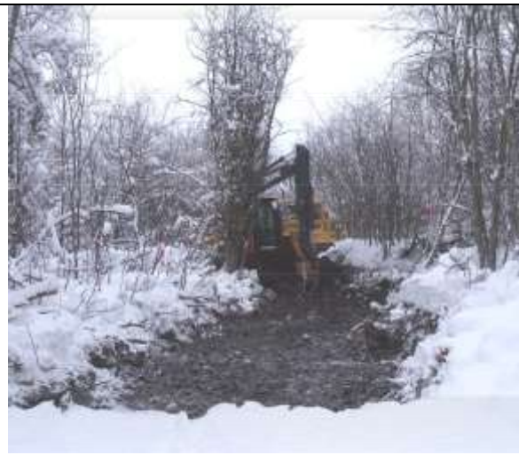
Photo 12. The excavator removing snow and topsoil from the historic channel.
