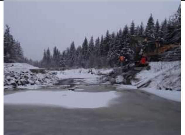
Photo 10. Beam Bridge abutments installed.
