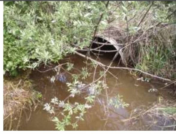
Photo 8. Outlet of main culvert at the Larson Rd Crossing, June 07, 2011.
