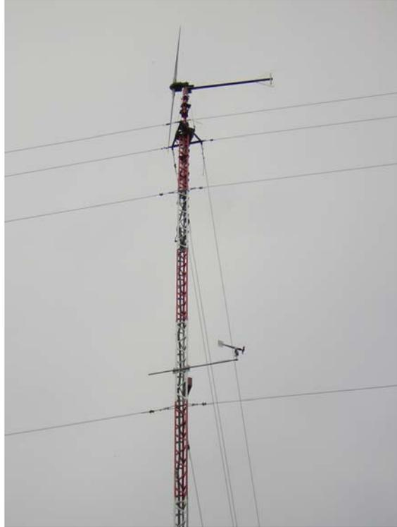
**Figure A3.3** Wind monitor on Nechako Lodge tower (on cross bar), 2005. Note the 3 kW wind turbine (Southwest Wind Power Whisper 175, 24VAC) at the top of the mast.
