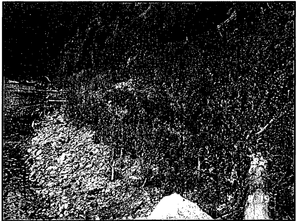
Plate 4.5.1-3: Example of wattle fencing used to stabilize areas of local erosion or sediment production.
