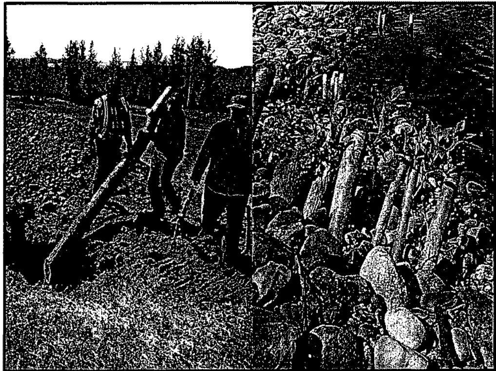
Plate 4.5.1-1: Example of live palisade construction to protect bank areas from erosion (photos by Dave Polster, R.P.Bio.).
