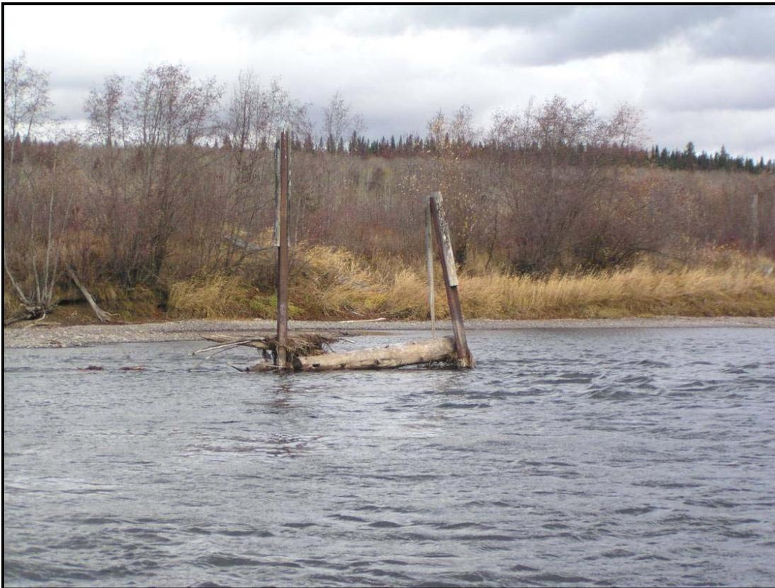
**Plate # 1. Date:** October 31, 2006. **Comments:** Showing the condition of the structure during the fall of 2006. Note the angle of the leading rail, and a lack of captured debris.
