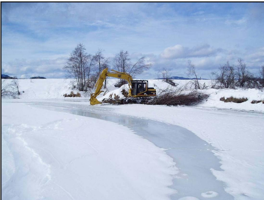
**Plate # 4.** **Date:** December 21, 2006. **Comments:** Showing the excavator perched on top of the woody debris, crossing out onto the ice.
