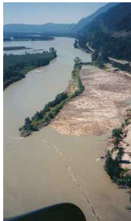
The Fraser River wood debris trap helps keep the Fraser safe for navigation.
